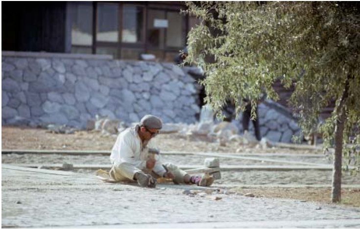
Workman adding non-skid surface to smooth cement
