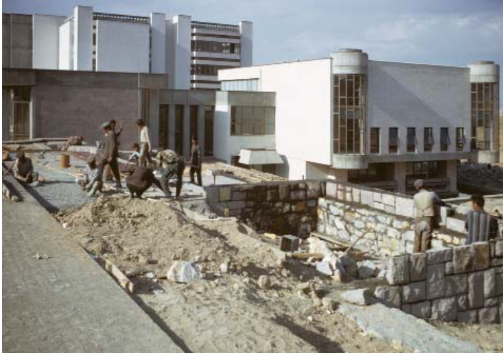
Workmen building the stairway next to the Library Building
