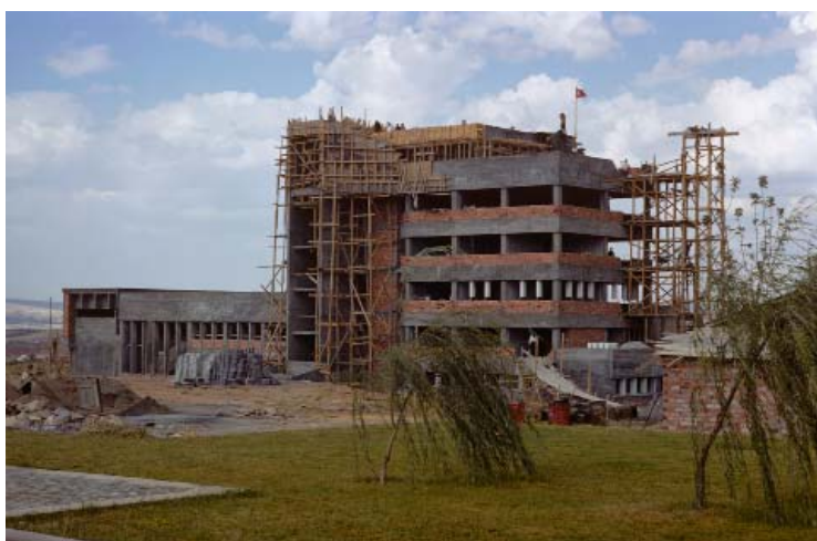
Constructing the Administration Building at METU
