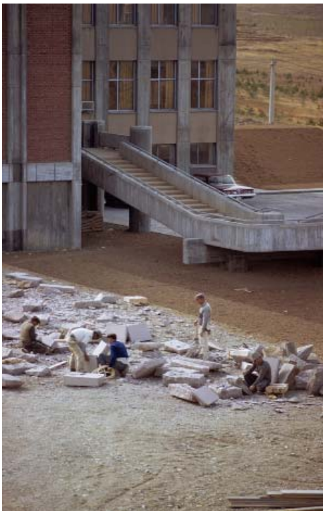
Masons working stone at METU
