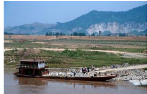
Rocks being unloaded from barge
